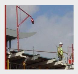
Higher Safety have been training large numbers of form-workers in the correct use of the Alsipercha (hangman). This has become the most popular safety solution for top down decking. Training details are available at Higher Safety.
